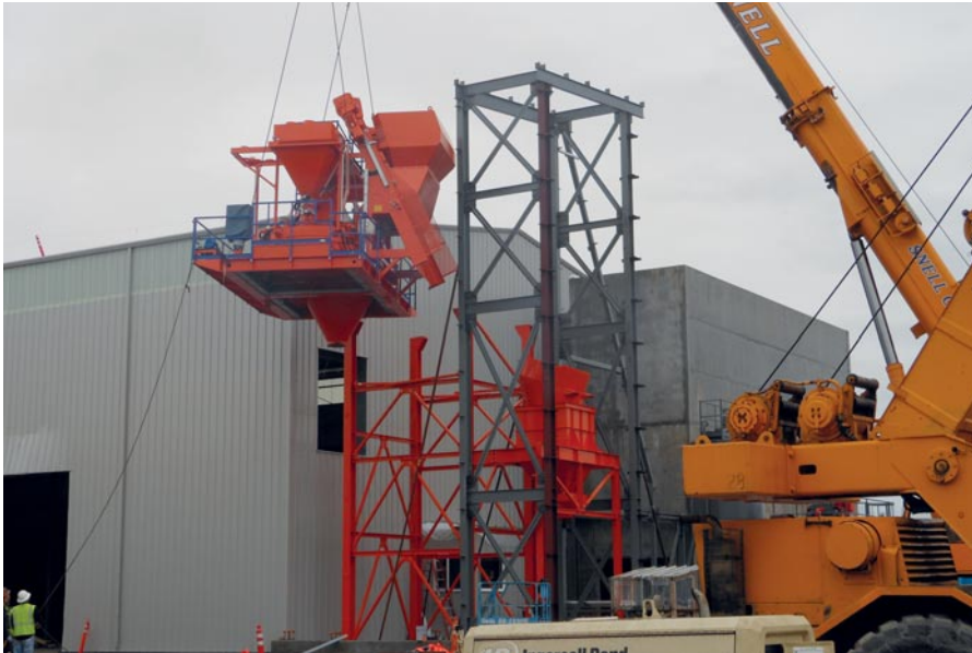
Figure 2: Under construction. The new ACT MobilMat Mo4500-5-PCS batching solution is positioned to feed EnCon's new tunnel segment production line as well as its preexisting precast retaining walls, median barriers, sound barrier panels, and commercial wall panel production lines. The new batch plant arrived from the Wiggert factory pre-assembled, pre-tested, wired and plumbed (air and water). One of the two cement silos shown here is dedicated to Portland Type 1 cement, and the other silo is split with one side containing silica fume and the other ground-granulated blast-furnace slag (GGBFS).
